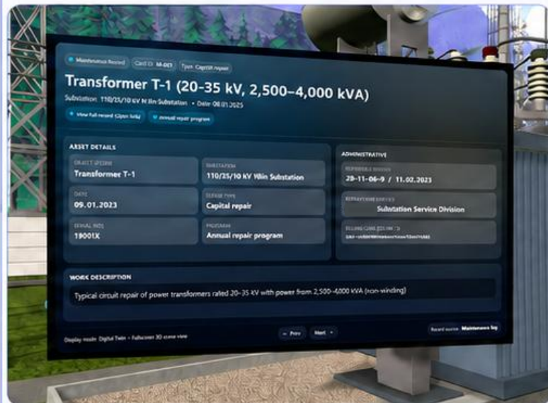
Transformer repair record
